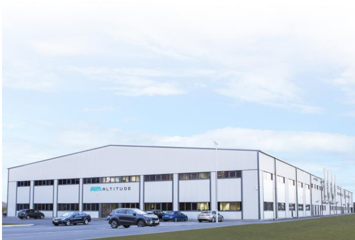
AIM Altitude's new facility at Bournemouth
